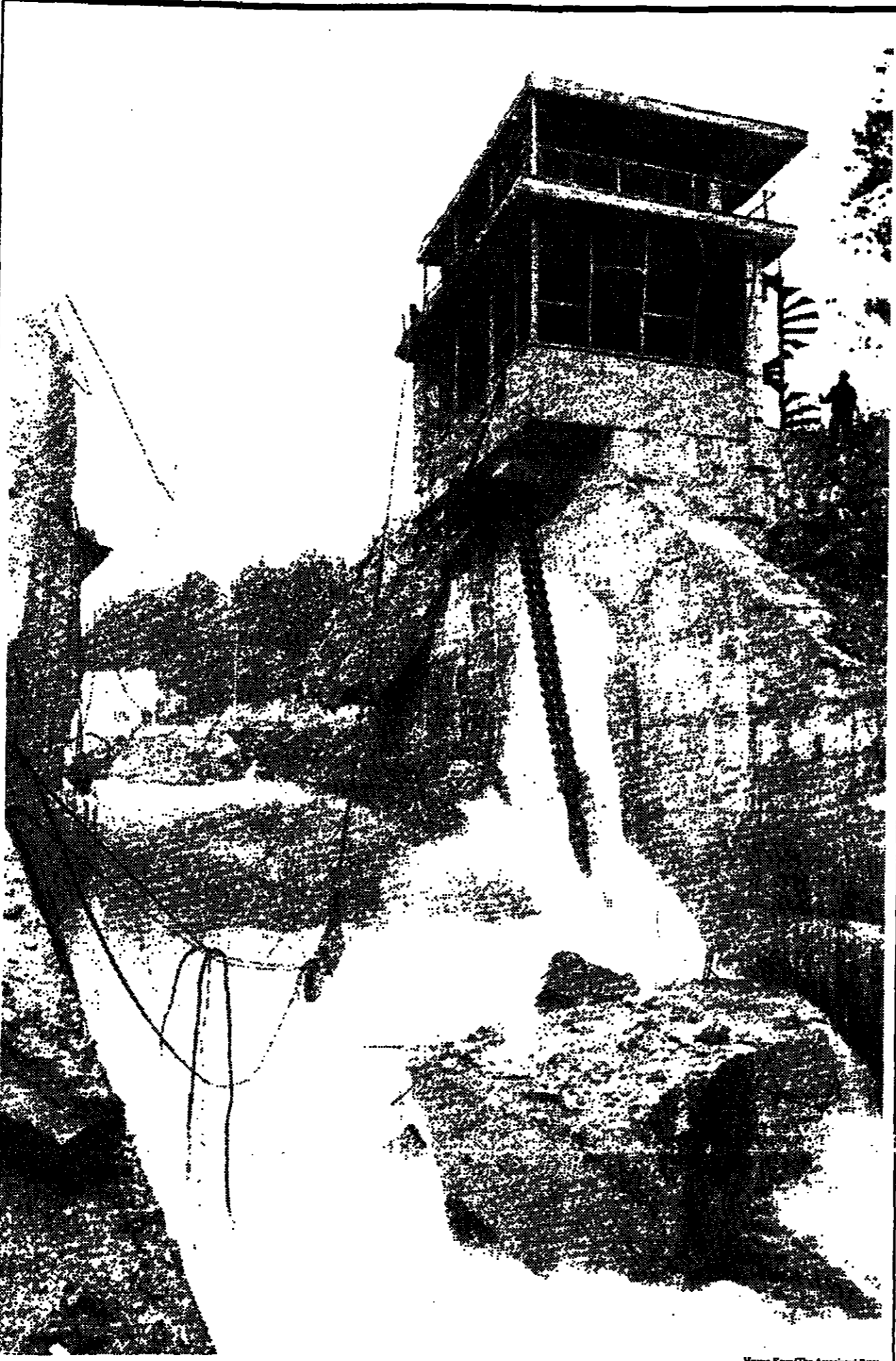
Rubble from a destroyed sluice gate lying in a spillway of the Peruca dam in Croatia, which was blasted by Serbian forces.
